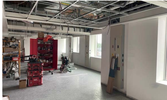
Pictured above are the North wing recovery rooms where the head wall units have been installed and the ceiling grid is almost complete.
