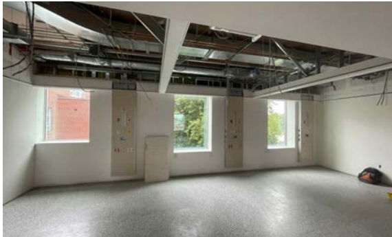
Pictured above are the North wing recovery rooms where the head wall units have been installed and the ceiling grid is almost complete.
